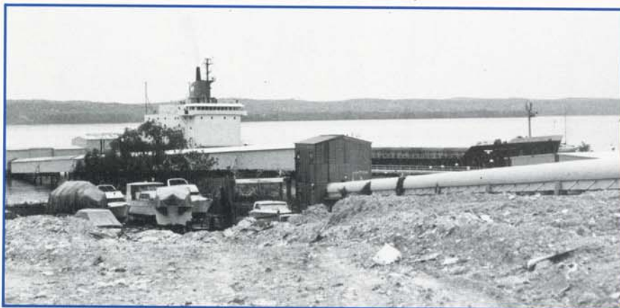
GYP SUM ROCK ORE FROM CANADA IS being unloaded (in the photo at left) from the large ore ship docked at its Hudson River berth, about one mile from U. S. Gypsum's Stony Point plant. A covered, conventional flat belt conveyor (seen exiting at the right of the picture) transports the gypsum ore from the ship to the rock ore storage shed for start of the manufacturing process.
