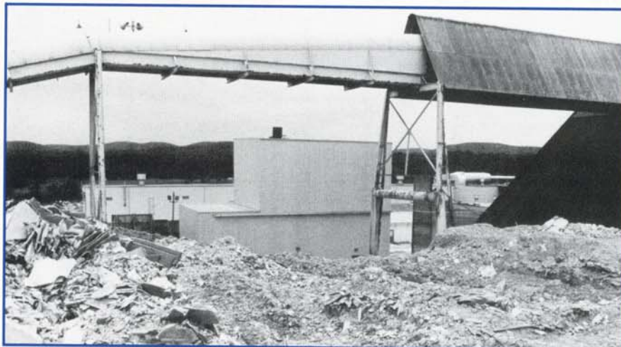
THE SERPENTIX CONVEYOR AT Stony Point is located at ground level on the corner of the waste processing building. The conveyor is seen here making its helical turn to the right and entering the building after elevating gypsum from the sizing hopper at its left.
