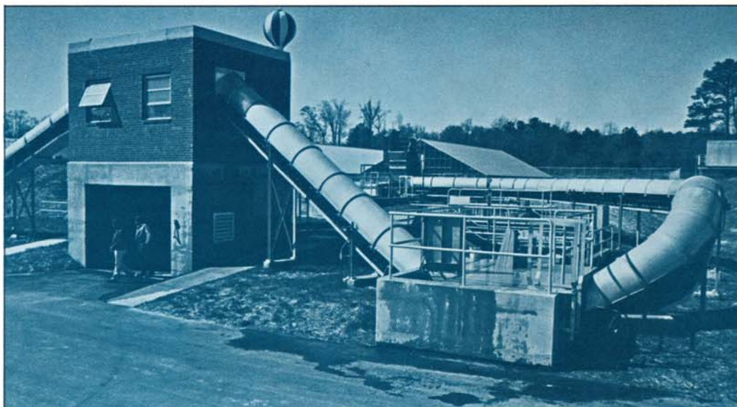
AFTER RECEIVING SCREENINGS (center, background) the longest Serpentix dips down (foreground) to receive collected grit. It then climbs sharply to discharge its load in the new collection building. A second Serpentix enters the building from the other side.
